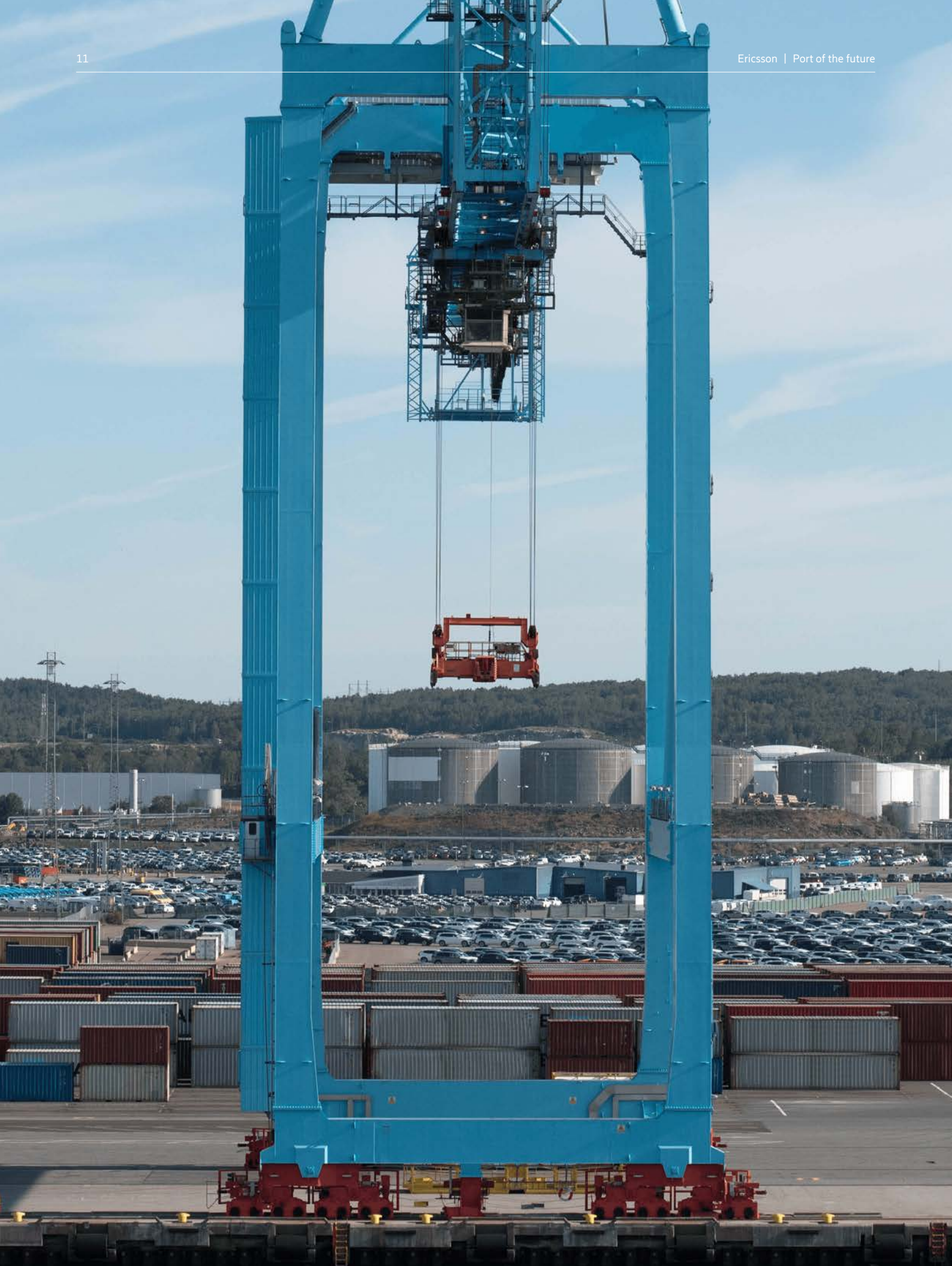
Container terminals handle the movement of containers in the port
