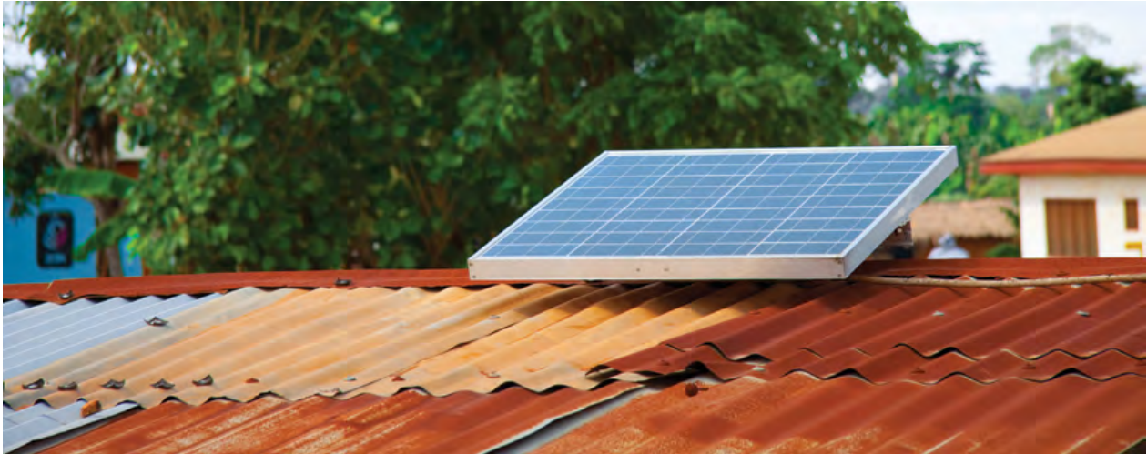
Rooftop solar panel in Ghana.
