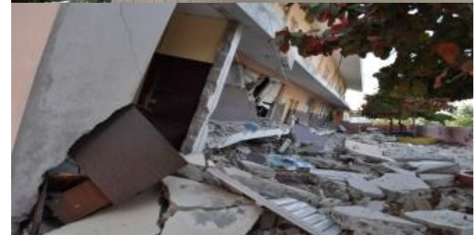
Figs: Haiti Damage Assessment, Hillside Settlements and High School Building
